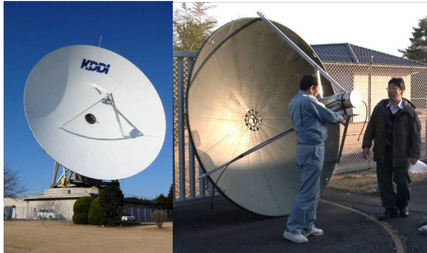
Fig. 7. 32m-diameter KDDI Antenna System IBA-4 and 23cm band feeding system assembly (septum feed+dish)
