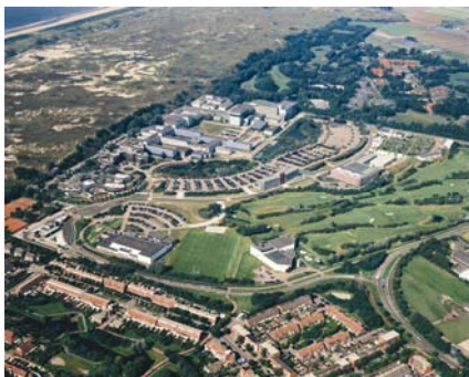
Fig. 1. Aerial view of ESTEC
