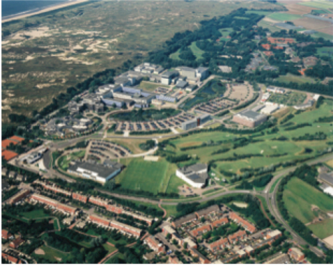
Fig. 1. Aerial view of ESTEC
