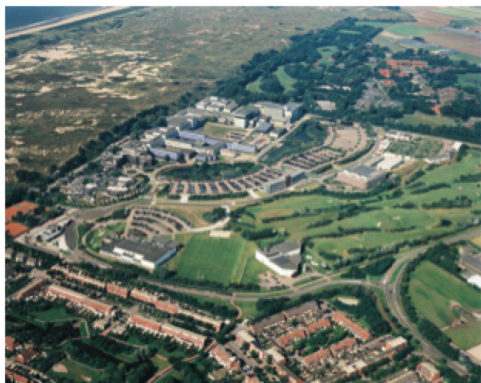
Fig. 1. Aerial view of ESTEC
